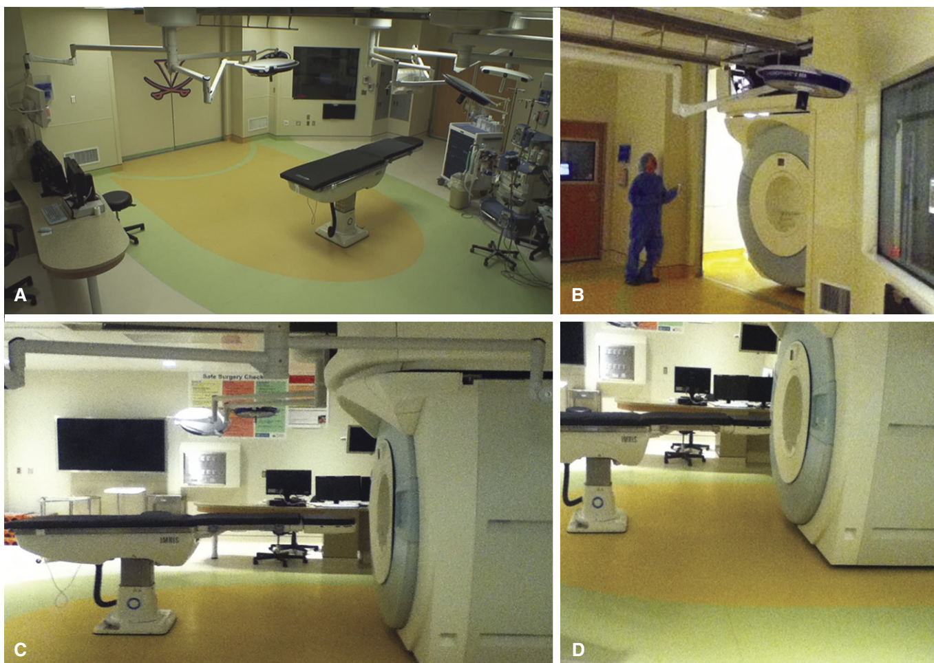
Fig. 5.8 Intraoperative magnetic resonance imaging (MRI) suite showing patient gantry in the operative suite (A). The magnetic bore is brought in from its resting “bay” for scanning (B). The movable magnet is ready to scan the stationary patient (C,D) during surgery and once that is done is sent back to its “bay”. Note the yellow colored area refers to the 5-G line where only the MR safe devices can be used.
